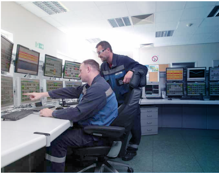
Monitoring and control at the Measurement Station
